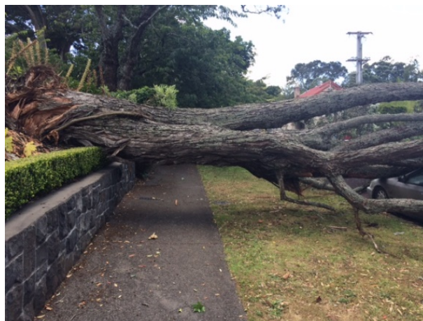
Fallen tree at Mt Hobson Water Pump Station
